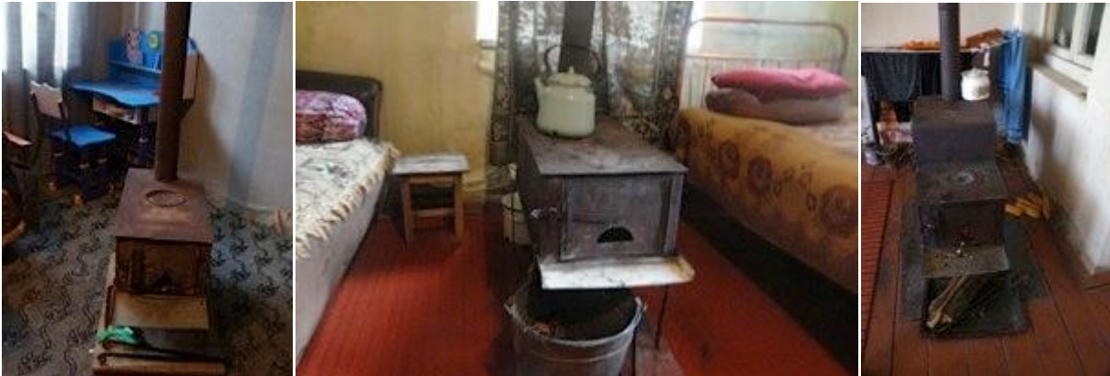
Figure 10 Typical application of heating stoves for space heating.
