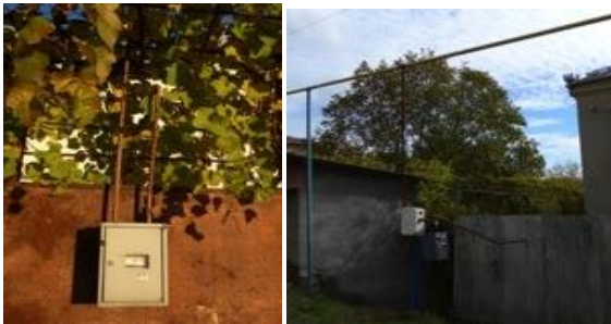
Figure 17 Examples of gas grid connected gasometers.
