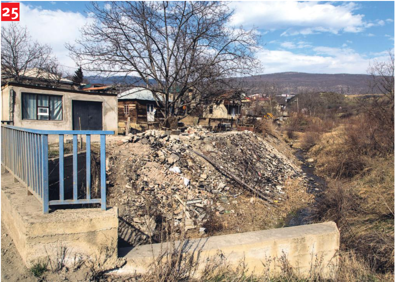
Photo 25, 26, 27: Within the limits of the Gldani housing complex, some sections of Khevdz mari River are enclosed in underground water tunnels. Intakes of the tunnels are not properly maintained and in some cases, adjacent areas are used for illegal disposal of waste causing the impoundment of water and swamping.
